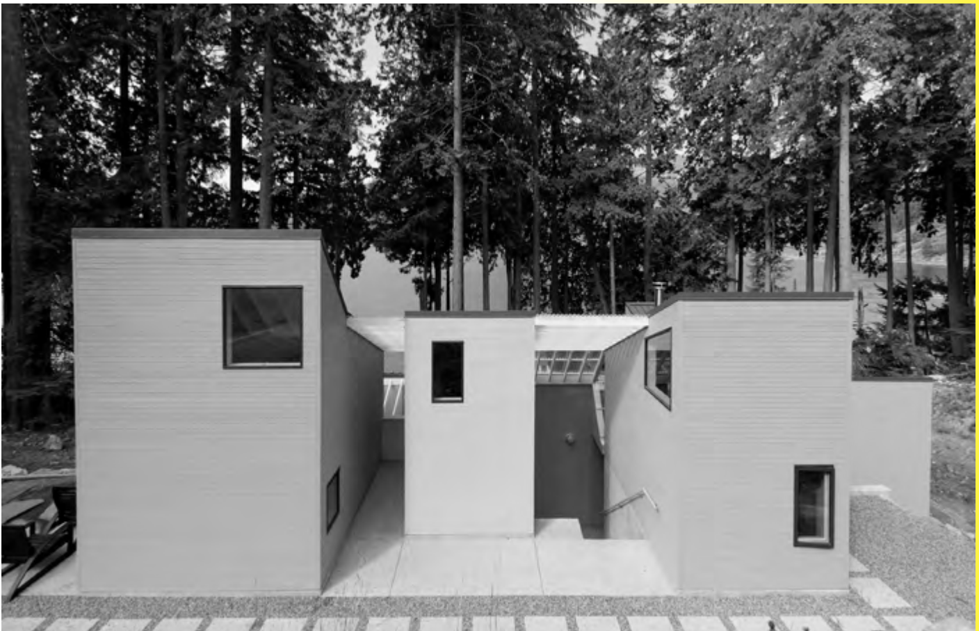
Simcic + Uhrich Architects' Gambier Cabin , Gambier Island
