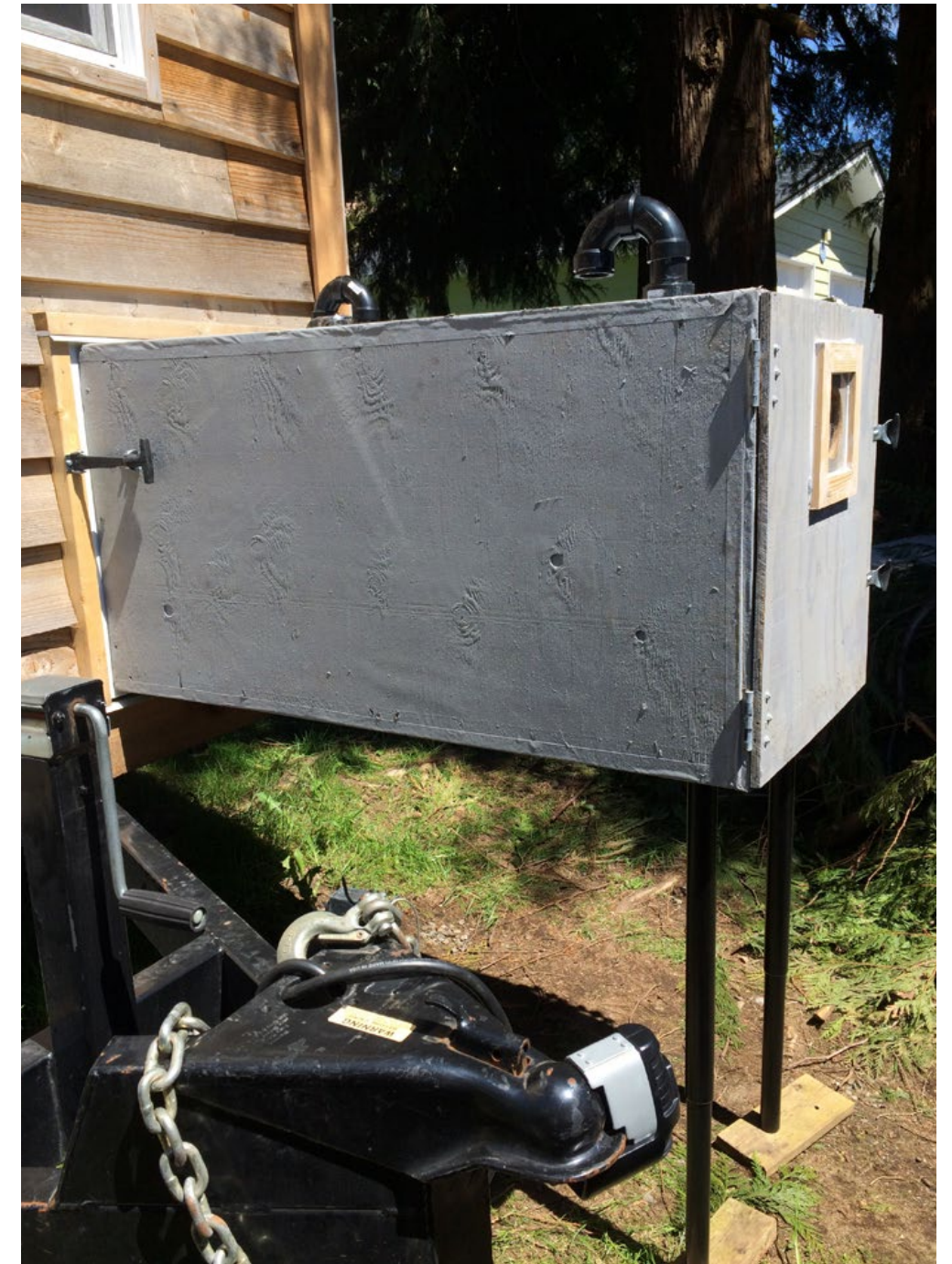
Solid waste catchment container for the Ecodomeo compost toilet model on a tiny house exterior.
